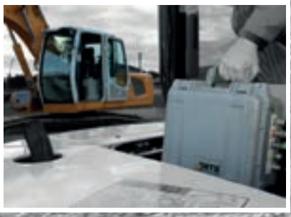
...on the excavator
