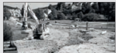
The "real" construction site
