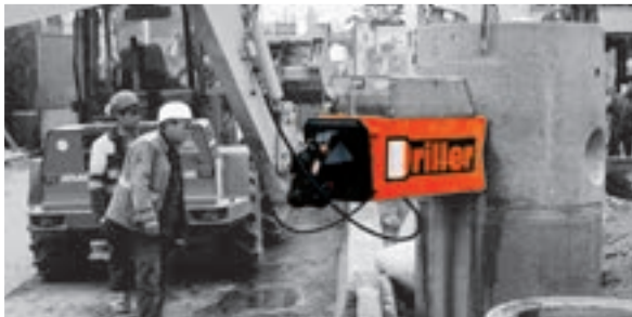
Horizontal shaft drilling
